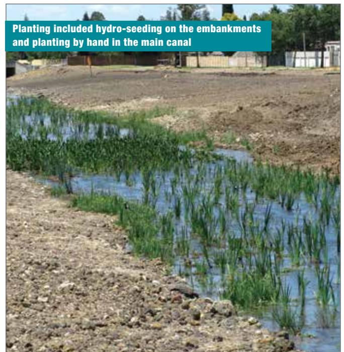
cluded providing reed beds and riffle sections for suitable habitat features to increase biodiversity, while stabilising the central stream and embankments with vegetation.
