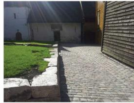
Permeable pavement and adjustment of the terrain surface stimulates local infiltration of storm water runoff. On the left hand side, green swales are visible that actively store and infiltrate rainwater. Photo: Johannes de Beer, Geological Survey of Norway.
