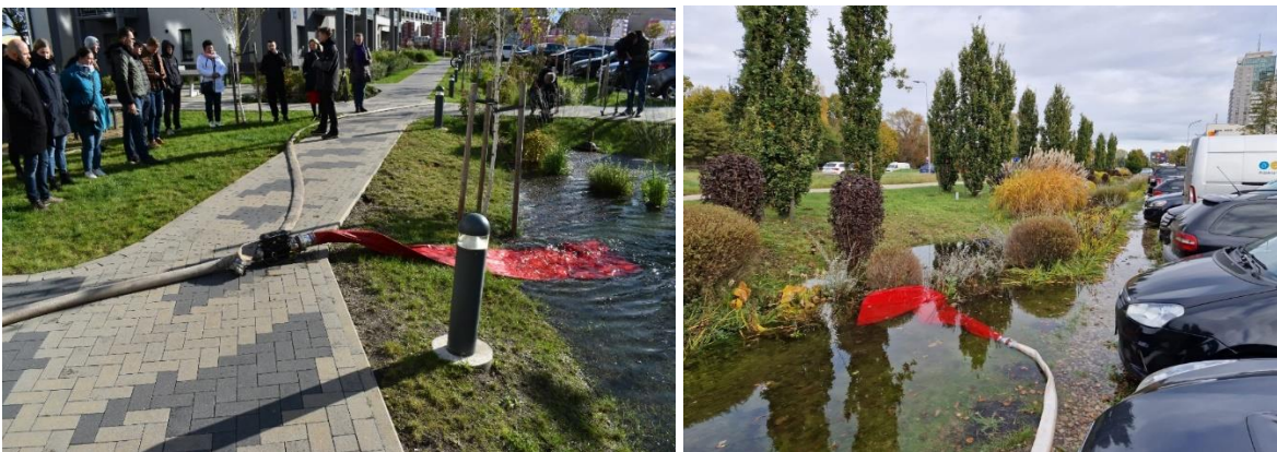
Figure 3. Infiltration tests in bioswale 2 and 8.
