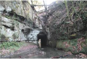
Fig. 1 – The Etruscan Ponte Sodo, a tunnel about 75 m long. It is a good example of the Etruscan hydraulic technology; its main purpose appears to have been to control floods and reclaim land close to Veii, the Etruscan city located a few kilometers from Rome (photo by Walter Dragoni).
